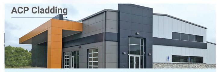
The aluminium composite panel is a composite material in which thermoplastic polythene core and the fire-retardant core material are sandwiched between two thin aluminium sheets. Polythene is not a fire-resistant material actually, it ignites and spread the fire.
