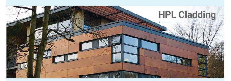
High Pressure Laminate (HPL) panels are a form of cladding typically manufactured by layering sheets of wood or paper fibre with a resin and bonding them under heat and pressure.
